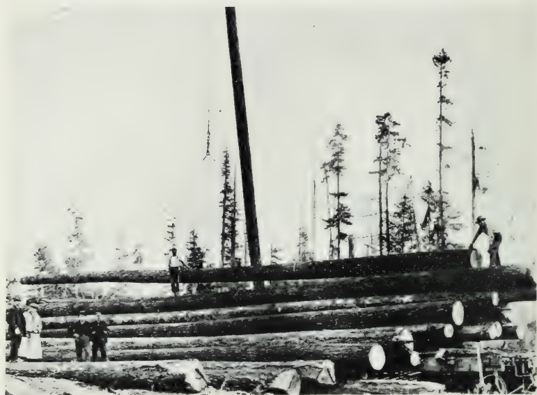
FIG. 55. OVERHEAD SKIDDING : LOGS ARRIVING AT HEADSPAR : BRITISH COLUMBIA.
